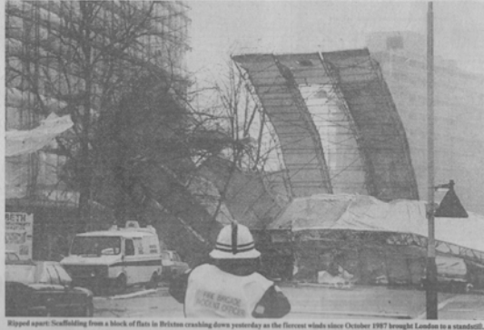
Shipped apart: Scaffolding from a block of flats in Belston crashing down yesterday as the fiercest winds since October 1987 brought London to a standstill.
